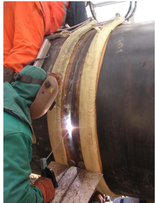
SHG used to power flexible induction blankets used for welding pre-heating
